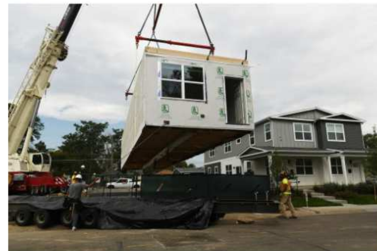
A crane stacking four 15-foot-wide, 60-foot-long modular-home segments to make a new duplex in Aurora, Colorado.
